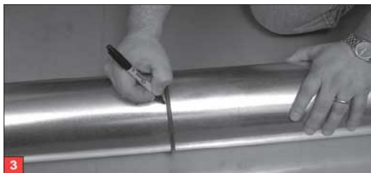
Mark pipe for cutting
