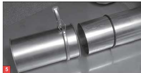
Put O-ring on cut pipe and slide slip joint over cut end
