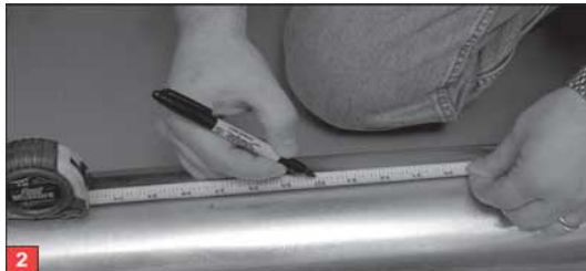
Mark approximately 4" less than required length
